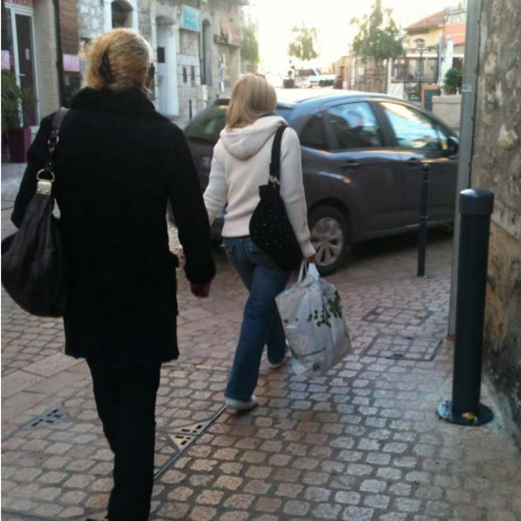
Figure 2: Example of a Passive Infrared Sensor installed within the large black pole next to the building wall. Source: Eco-Counter, n.d.
