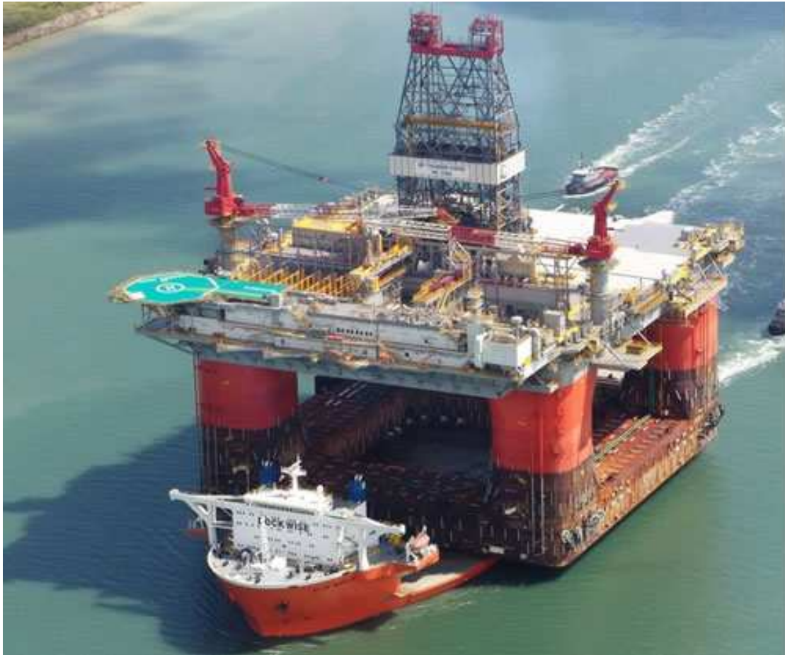
Figure 2.4: Semisub Drilling Rig en Route to new location. To better appreciate the size of this drilling rig, note the size of the 6-story building on the deck of the carrier vessel towards the front of the carrier ship.
