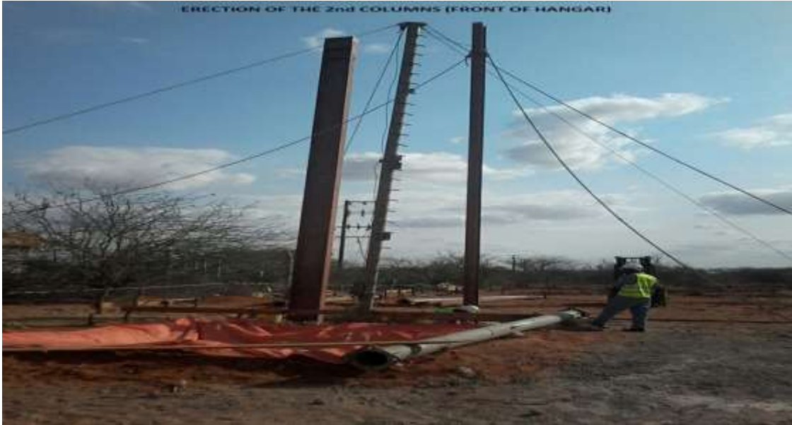
Manually Operated Derrick cranes being used to erect structural steel members
