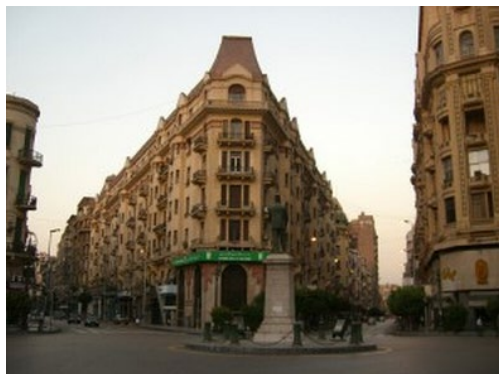
The Yacoubian Building, No. 34 Talaat Harb, Cairo, Egypt
