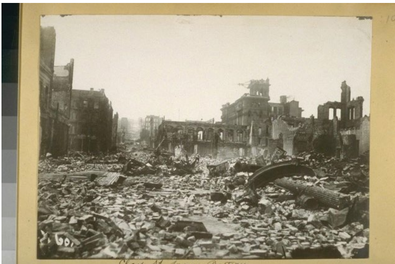
Destruction on San Francisco's Clay Street after the 1906 earthquake (UC Berkeley, Bancroft Library)
