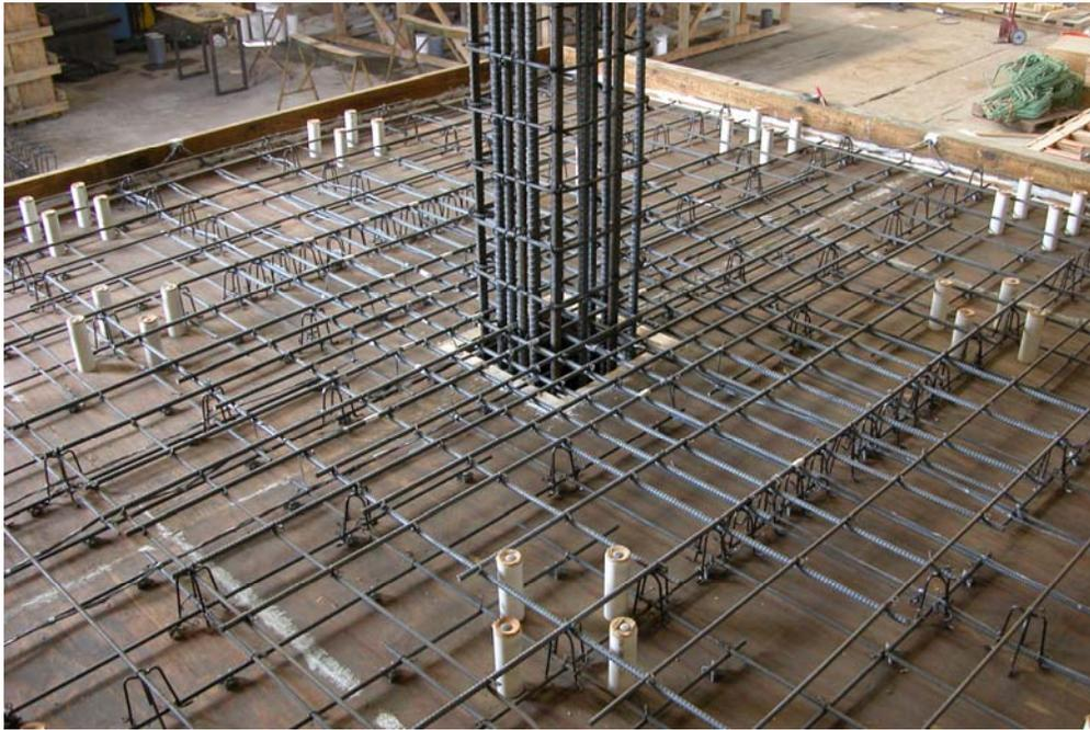
Figure 2.28: Steel cages and slab forms (Specimen LG1.0).
