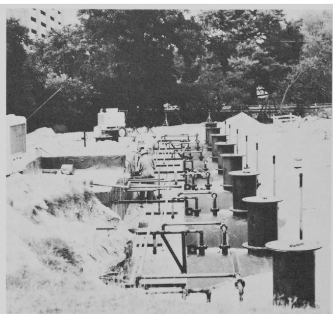
Fuel-oil storage is under construction at many locations throughout the state in 1973. These projects are characteristic of the energy crisis of 1972-1973 and symptomatic of the transition to a new energy economy. Increased fuel-oil storage is a requisite of natural-gas curtailments. Most of this energy is used for production of electric power and process and utility steam. The tanks shown here will store 10,000 barrels of fuel oil.
