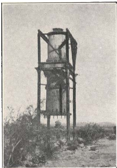
a. Furnace on the Cooksey Prospect. Said to have produced 75 tons of sulphur; built about 1900. The foundation of the furnace rests on Castile gypsum. Rustler Hills in the distance.
