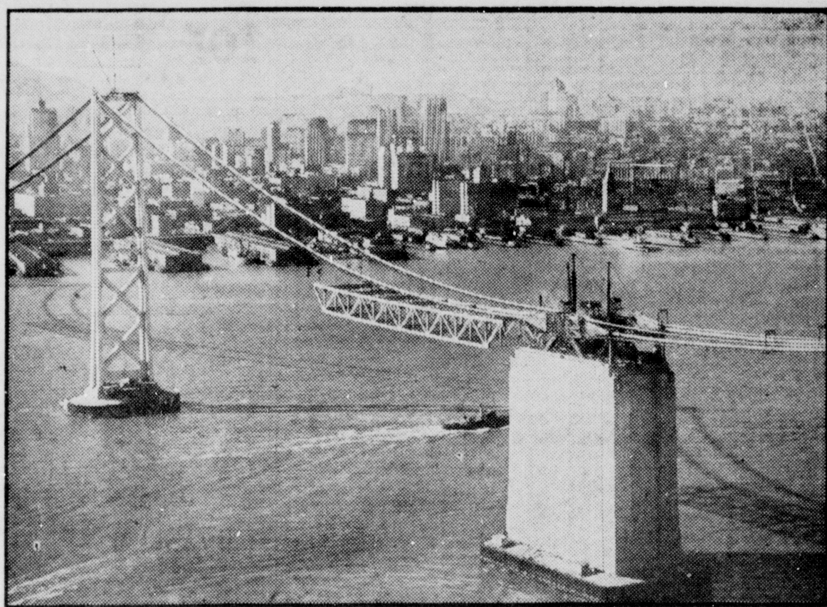
Rapidly, section by section, skilled engineers are assembling the mammoth San Francisco-Oakland Bay bridge, longest in the world. This photo, taken from the air, shows the newest phase of construction on the 4 1/2-mile long span—trusses which form the deck of the bridge—in
