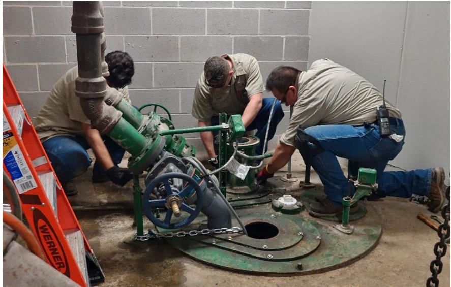
Technicians work on sump pump at the Texas Swim Center.
