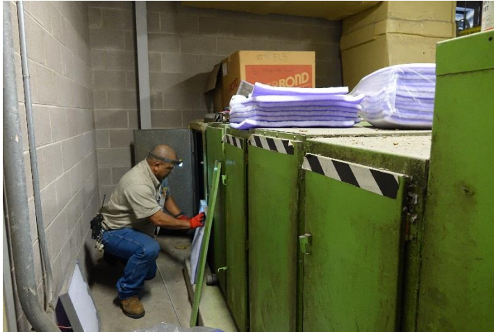
Technician changes filters on air handler unit.
