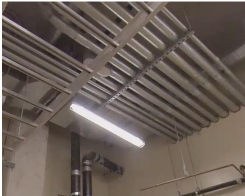
Figure 7: Electrical conduits that preventing the accessibility to the air handling unit.
