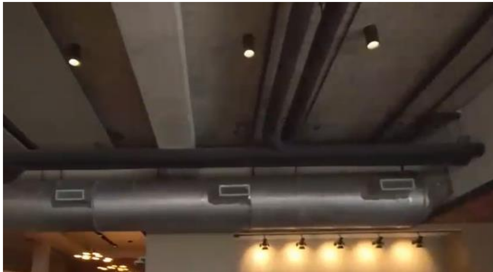
Figure 8: The lighting from light fixtures is blocked by an HVAC duct.
