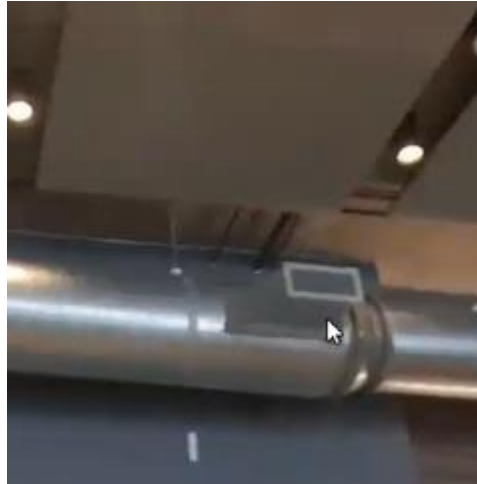
Figure 10: Ceiling fabric system moved away from the hangers.
