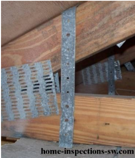
Figure 12: Roof Wall Connection Strap Example
