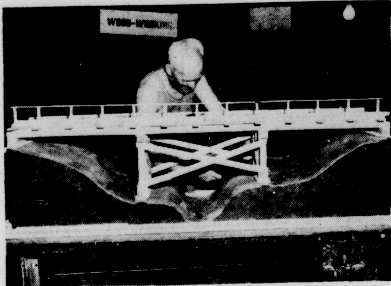
BUSMAN'S HOLIDAY was taken by Sergeant Joe Glenn when he built the model trestle bridge that the Army ROTC will use this fall. Of semi-permanent nature, the bridge required sixty man-hours and $40 worth of raw materials.
