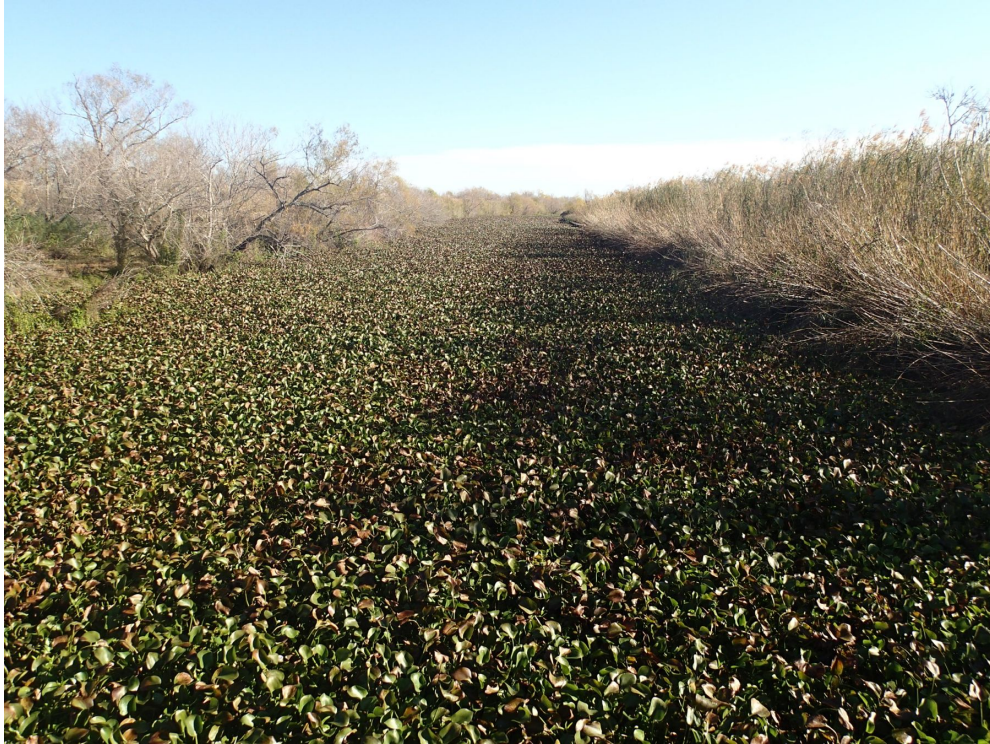
Figure 10. Downstream view of diversion canal from bridge that is accessible off TX-35 (wp04). Canal is completely choked by floating plants (appears to be water hyacinth). Photograph by Ben R. Hodges, ©2013. File wp004 bENE BridgeOverDiversionChannel i032.
