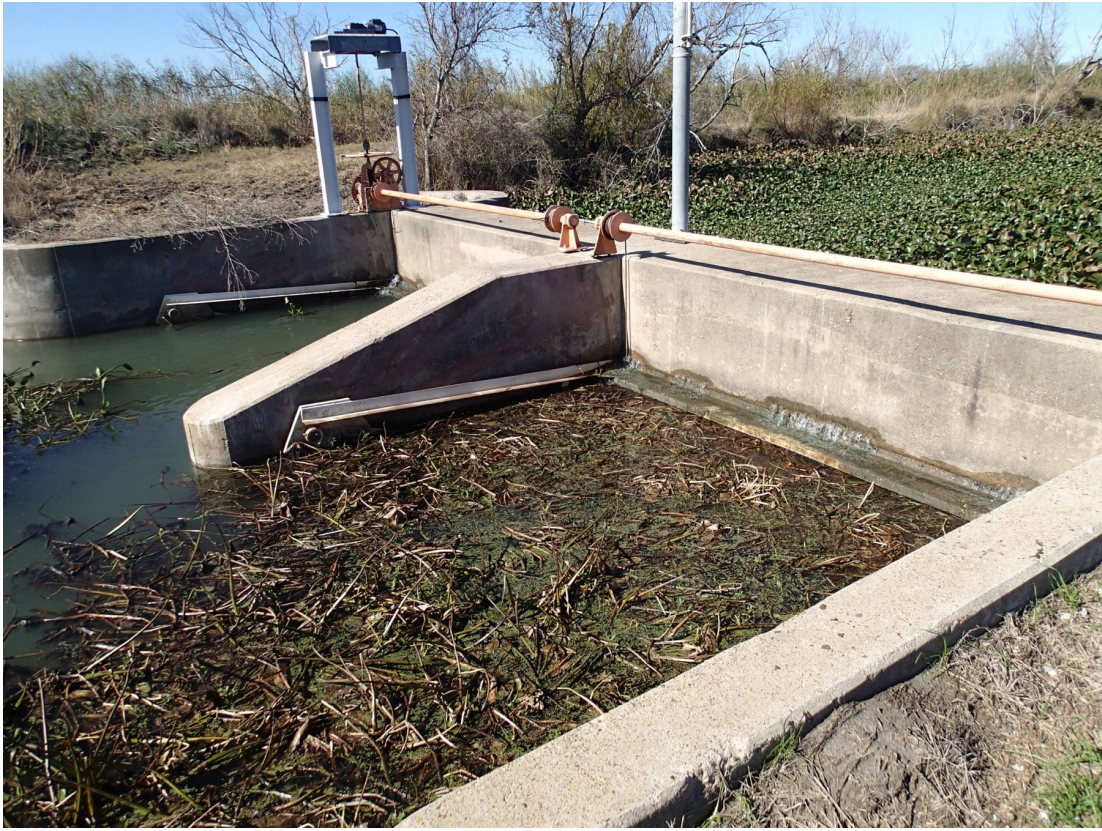
Figure 30. Close gates separating upstream and downstream sections of Goff Bayou at wp14. Photograph by Ben R. Hodges, ©2013.
