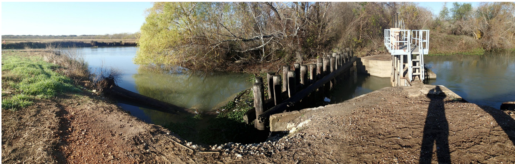
Figure 5. Diversion canal upstream of the saltwater barrier (wp03). Guadalupe River is to the left. Diversion canal flow is from left to right. Wooden pilings prevent river flotsam from clogging gates, which are part of concrete structure on right. Composite panorama photo using DoubleTake software distorts linear relationships. Photograph by Ben R. Hodges, ©2013. File wp003 bSWtoWNW UpstreamDiversionChannelGate p022to24.
