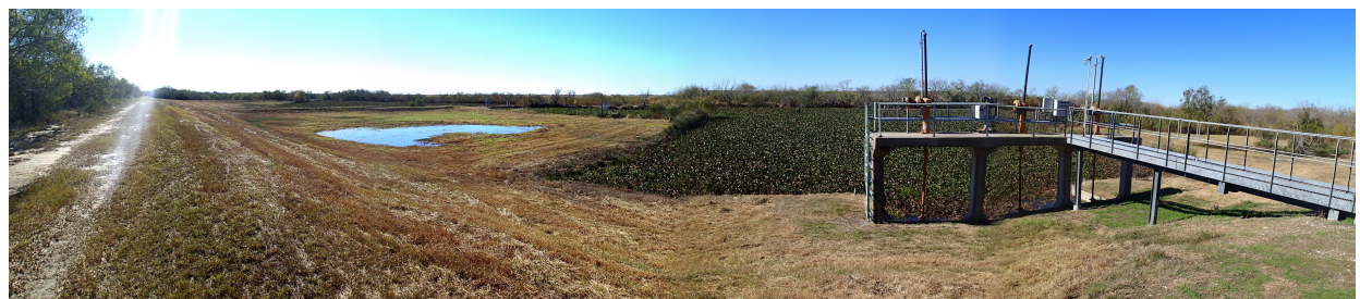
Figure 24. Panoramic view from south to west of Goff Bayou and the gates connecting the bayou to the industrial canals on the opposite side of the Victoria Barge Canal. Goff Bayou is entirely choked with floating plants (appears to be water hyacinth). In center of the photo are the downstream gates at wp14. Composite panorama photo using DoubleTake software distorts linear relationships. Photograph by Ben R. Hodges, ©2013. File wp013 bStoW GoffBayouGates p086to089.
