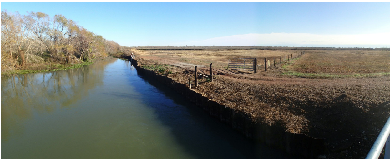
Figure 7. Freshwater diversion canal (wp03) looking downstream from gate structure. High banks require extreme flows to connect with the upstream reaches of Schwings Bayou. Composite panorama photo using DoubleTake software distorts linear relationships. Photograph by Ben R. Hodges, ©2013. File wp003 bNNetoS DiversionChannelFromUpstreamGate p028to030.
