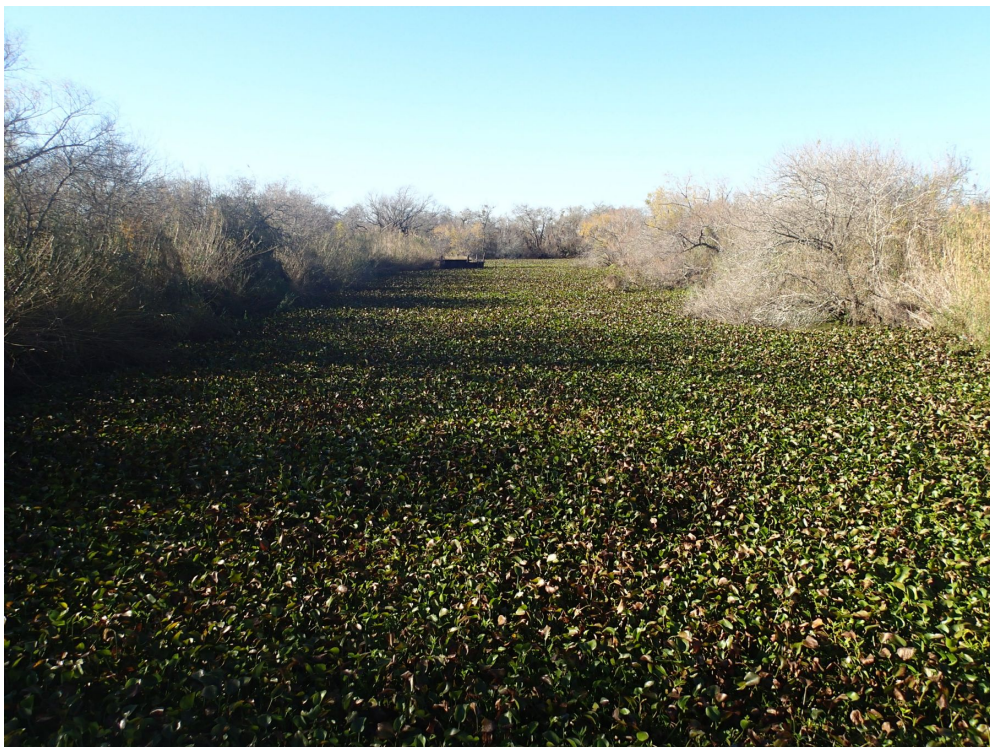
Figure 11. Upstream view of diversion canal from bridge that is accessible off TX-35 (wp04). Canal is completely choked by floating plants (appears to be water hyacinth). Photograph by Ben R. Hodges, ©2013. File wp004 bNNE BridgeOverDiversionChannel i033.
