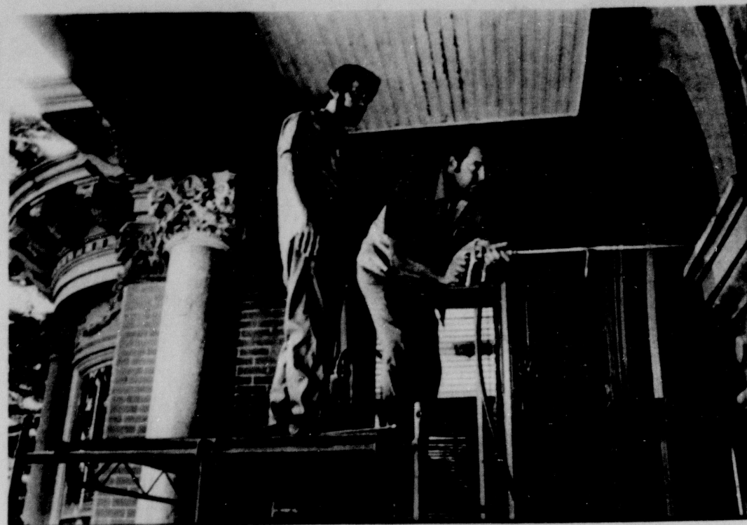
—Texan Staff Photo by Will Van Overbeek Facelift for an 84-year-old Ernest Strawser and Gerry Huff work on the front of the Littlefield Mansion with a high-pressure water cleaner. Built in 1893, the University landmark is receiving mortar work, recaulking, repainting and waterproofing.
