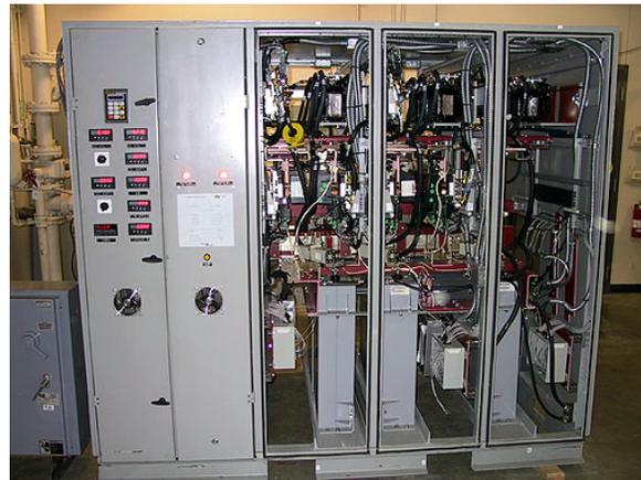
Figure 5. 2 MW continuous duty ARCP converter
