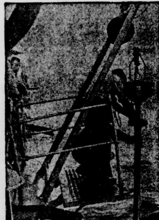
Penetrating the ocean floor with a "bottom corer." Analyses of bottom sediments contribute to undersea warfare as well as providing insight into the origin and evolution of our planet.
