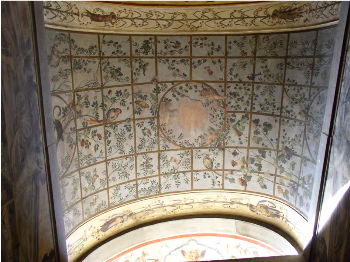
Fig. 6.8 Palazzo Vecchio, Florence, Marco da Faenza, painted pergola on the ceiling at the foot of the stairs leading from the Room of Leo X to the Quarter of the Elements (photo: author).
