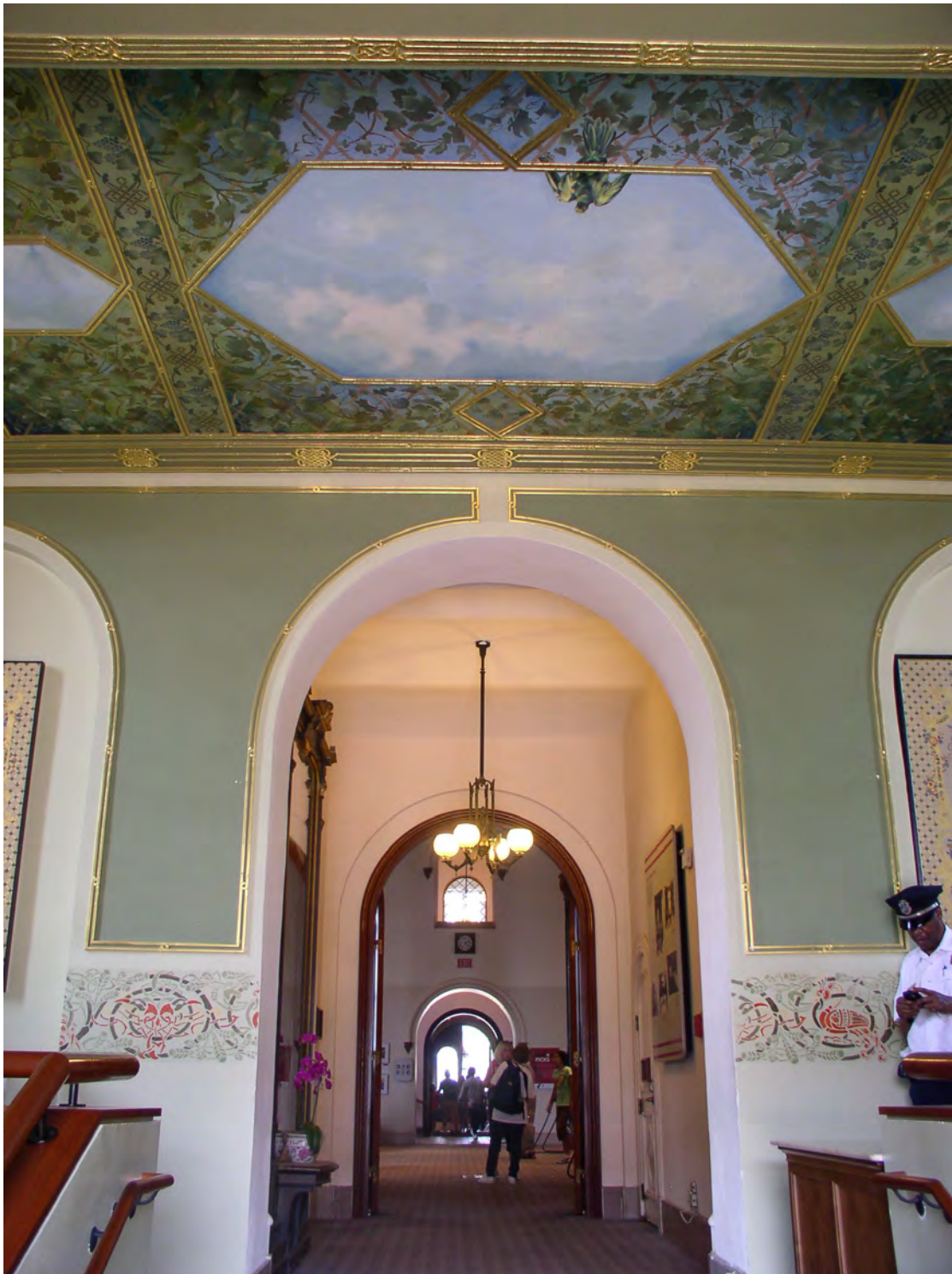
Fig. 9.5 Smithsonian Castle, entrance vestibule from the Enid A Haupt Garden. View of the vestibule with ceiling and wall decorations by Grace Lincoln Temple (1864-1953). (photo: author).
