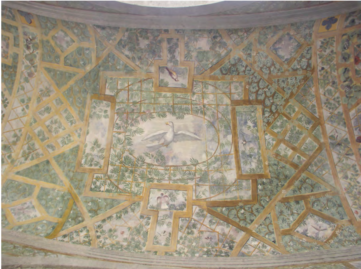
Fig. 6.51 Villa Farnese at Caprarola, circular portico, illusionistic pergola, section 2W (photo: author).
