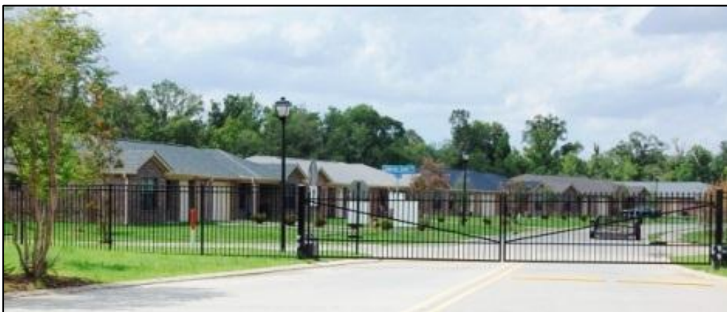
Figure 21: Senior Residences of Central entrance gate. Source: ProdiGem, L.L.C. (ProdiGem, L.L.C. 2011)
