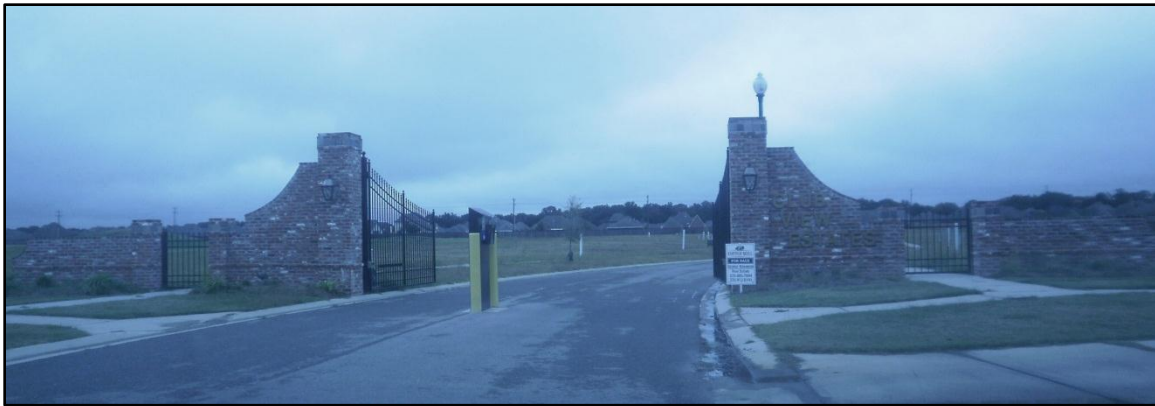
Figure 24: Entrance to Club View Estates
