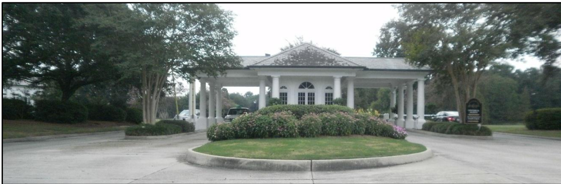
Figure 14: Front gate at the Country Club of Louisiana. Far right lane for residents with automated gate cards; right lane for visitors who must stop at guard house.
