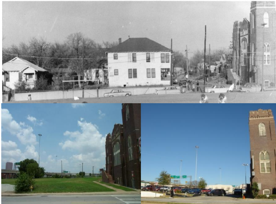
FIGURE 6-18. Three photos showing the west north/northwest side of the church over time: (a) St. Paul Neighborhood, mid-20 th century, cropped from Figure 6-17. (Photographer unidentified) (b) St. Paul Neighborhood in 2002 (UT Austin Field School), and (c) St. Paul Neighborhood in 2009 (Photo by Ibukun Saucer.)
