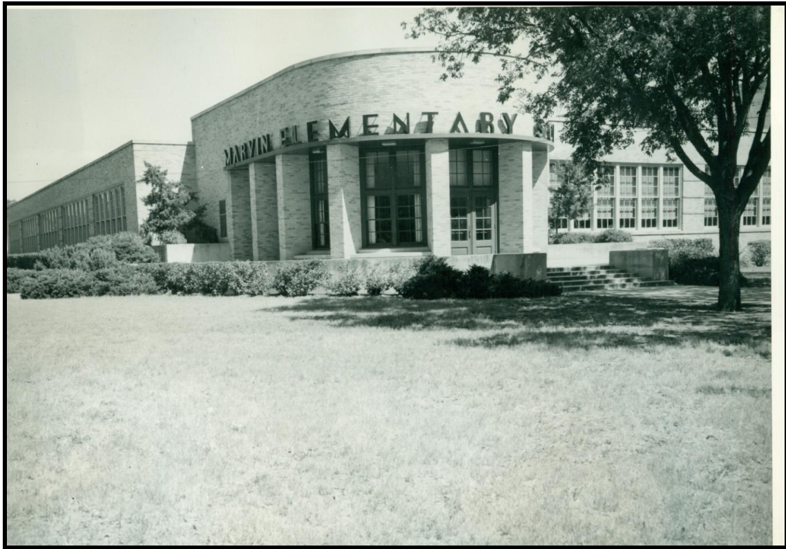
Figure 14. Addition to Central Ward campus, renamed Marvin Elementary, 1939.
