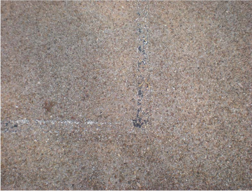
Figure 19: Basketball Court Painted Lines
