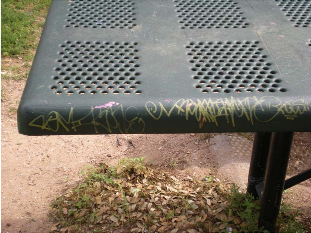
Figure 8: Park Bench at Civitan Park
