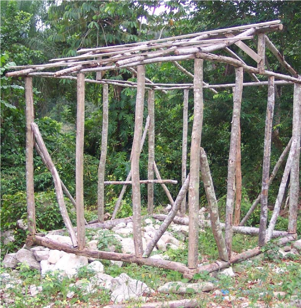
Figure 17: Construction of a Traditional Style House
