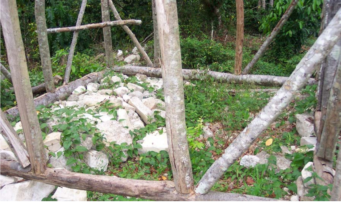
Figure 18: Close-up of Stone Foundation on Traditional Style House
