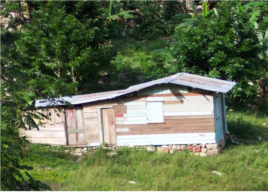
Figure 14: Modern House with Functional Stone Foundation
