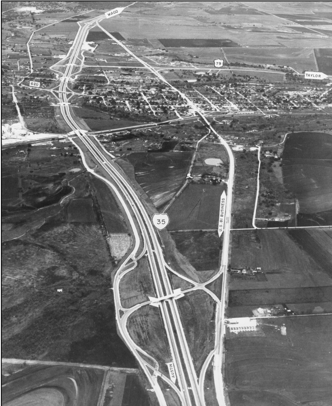
Figure 54: Interstate 35 not yet open at Round Rock, which lies in the background. Note how I-35 cut through part of residential Round Rock. Below the airplane, but not visible, is the FM 1325 exchange.
