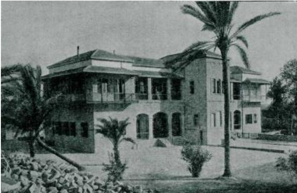
Illustration 1: New CMS Hospital building in 1907. 75
