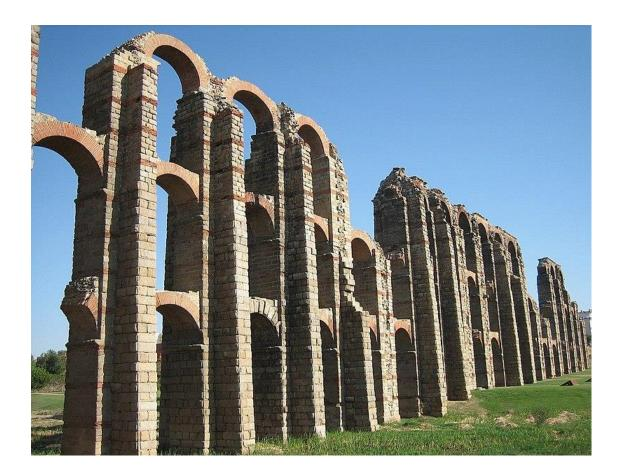
Figure 11: Roman Aqueduct at Merida (Acueducto de los Milagros), 1<sub>st</sub> century AD, Merida, Spain. Granite and red brick. 25 m high x 830 m long. Image: WikiCommons
