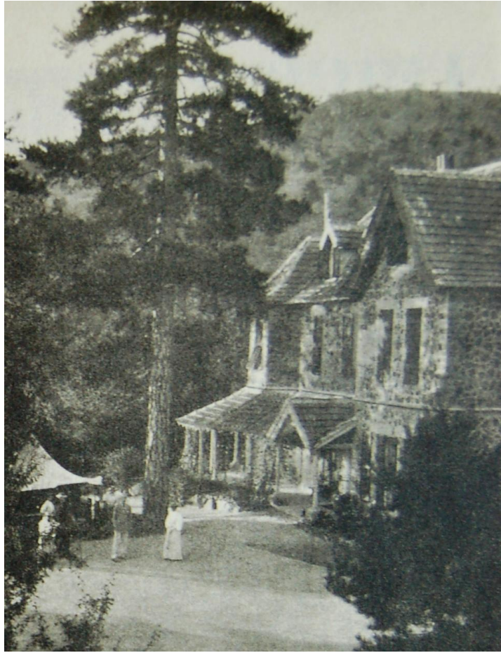
Figure 3.10. Stone house in Troödos.
