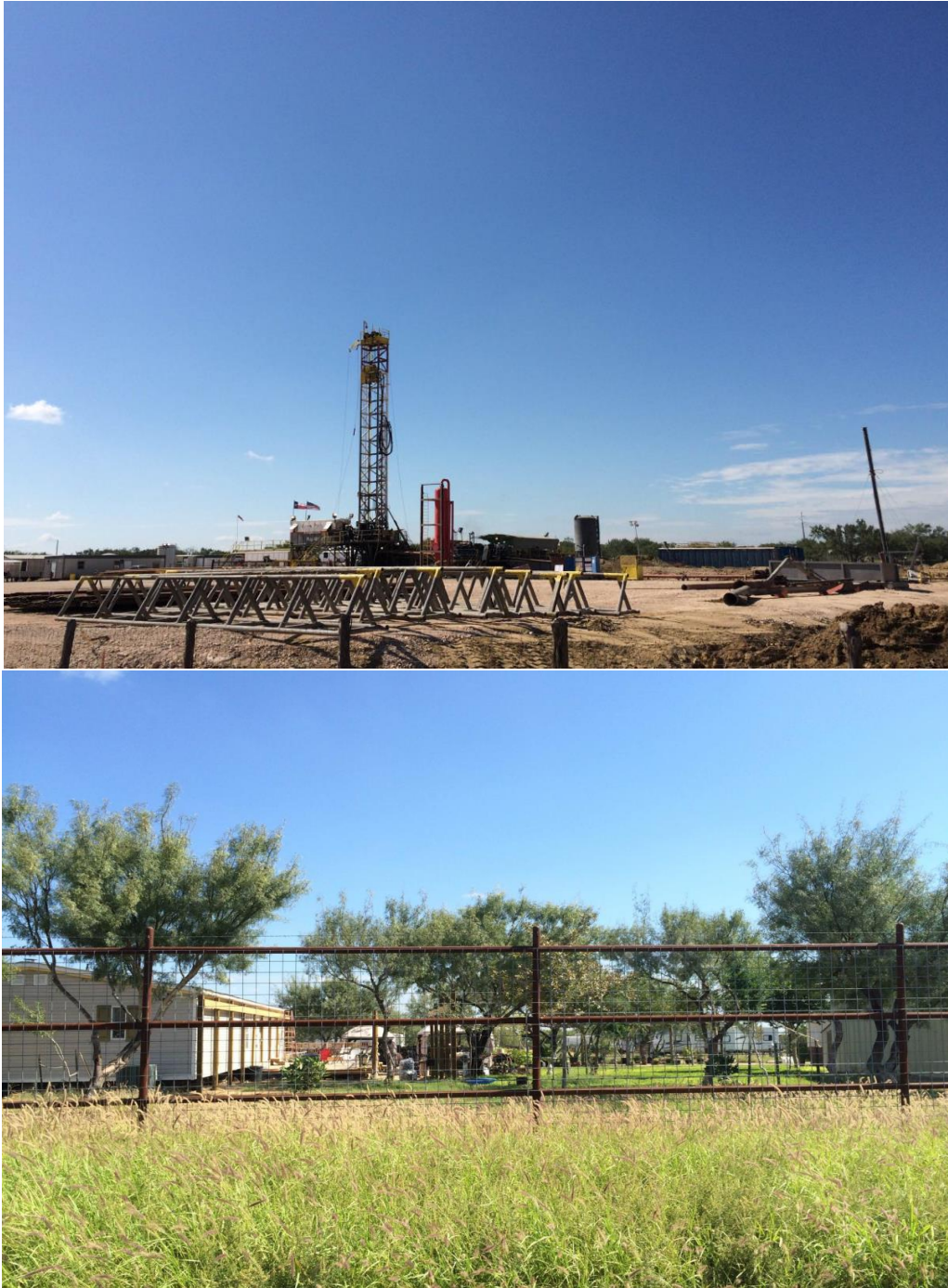
Figure 7.7. Well Pad in La Moca Ranch (colonia), Northwest Webb County, 2014 132
