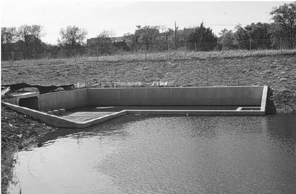
Figure 4.7 – Concrete Lined Detention Basin, City of Austin (Barrett, 1999)
