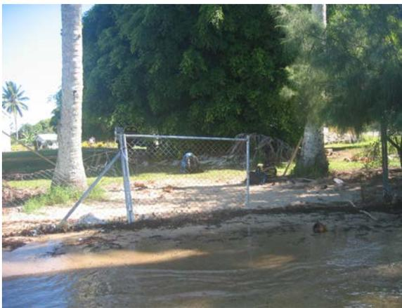
**Fig. 8. The fence along the shoreline at the hospital in Pangai, Lifuka Island is underwater during high tide. Coastal erosion is damaging buildings and infrastructure such as wharves and sea walls. 'Apai Moala visited this exact site in early June 2006 prior to our arrival and found high tide reaching behind the coconut trees which is about 1.5 to 2 m farther inland than when we visited in November 2007. This suggests that**
