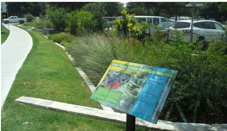
Figure 3. The rain garden outside of One Texas Center is an example of an engineered water quality control.
