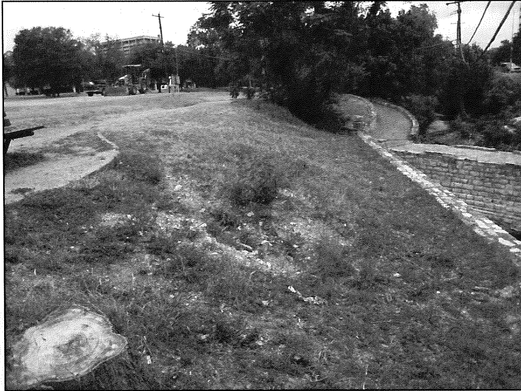
Figure 15. Walkways and stone retaining walls along Waller Creek.
