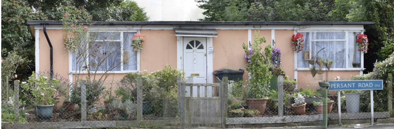
Figure 2 An Excalibur Estate Prefab. Photo from July 2017 by Hank Parker.
