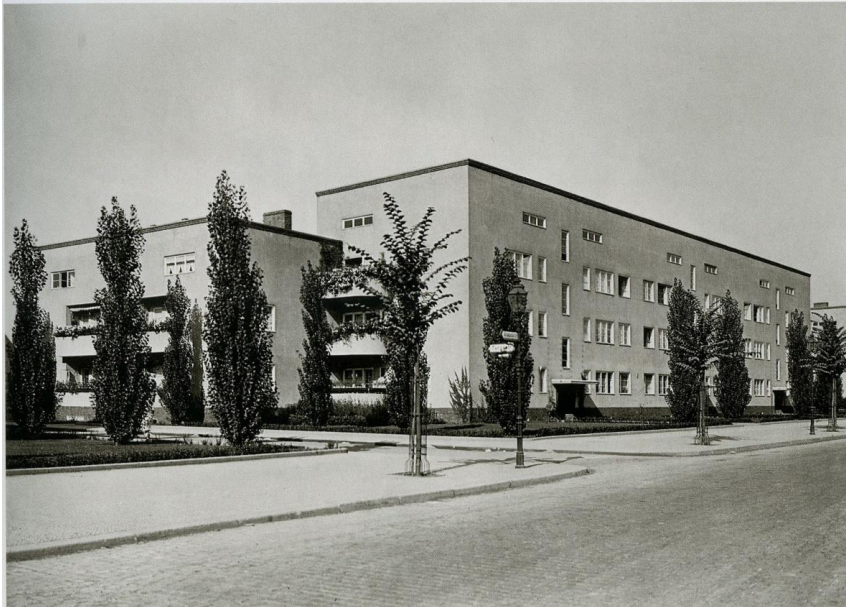
Figure 3.7. View from street, Afrikanischestrasse apartment building, 1925-1927. ( Mies in Berlin Fig. 86).
