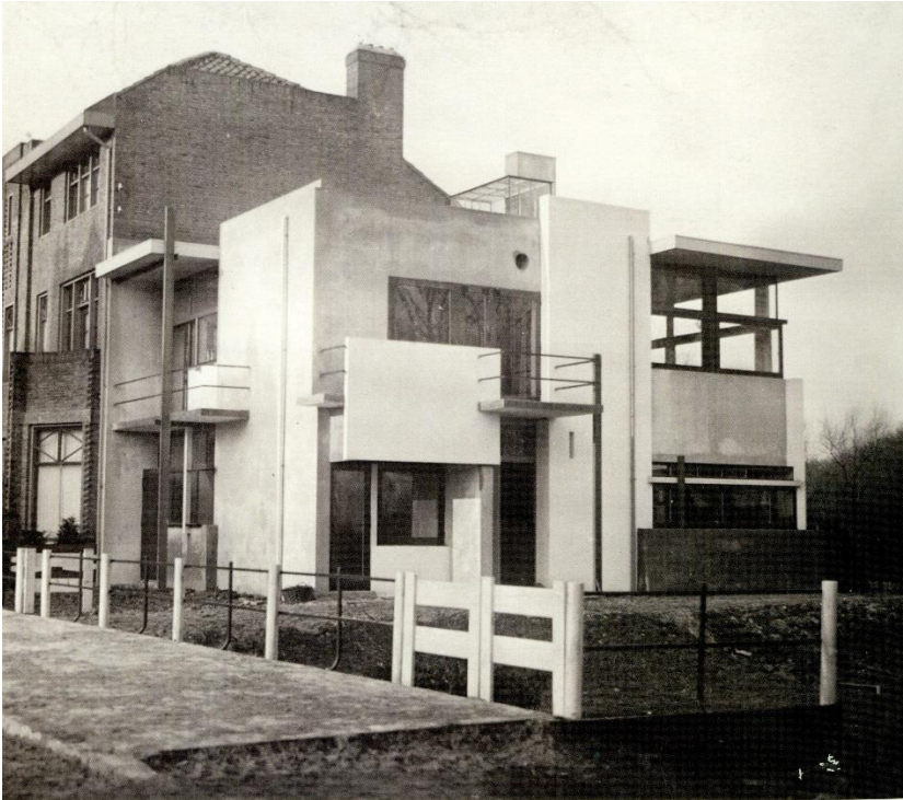
Figure 3.11. Rietveld Schröder house, view from the south, Utrecht, Netherland, 1924. (Iida van Zijl, Gerrit Rietveld [New York: Phaidon, 2010], 58)
