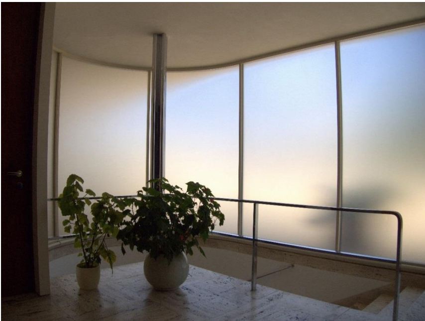
Figure 4.14. the frosted walls of vestibule, Tugendhat House, 1929 (Photographed by author).
