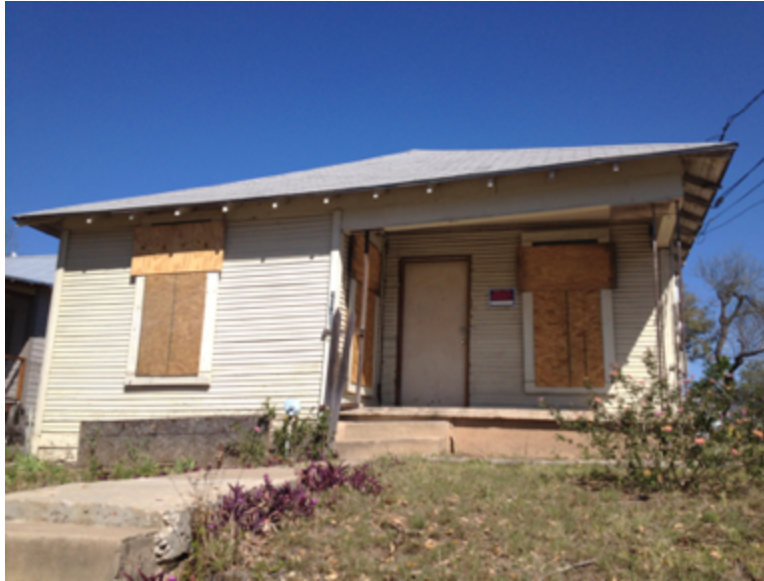
Figure 2: Abandoned home located at 2008 E. 13th Street (11-42).
