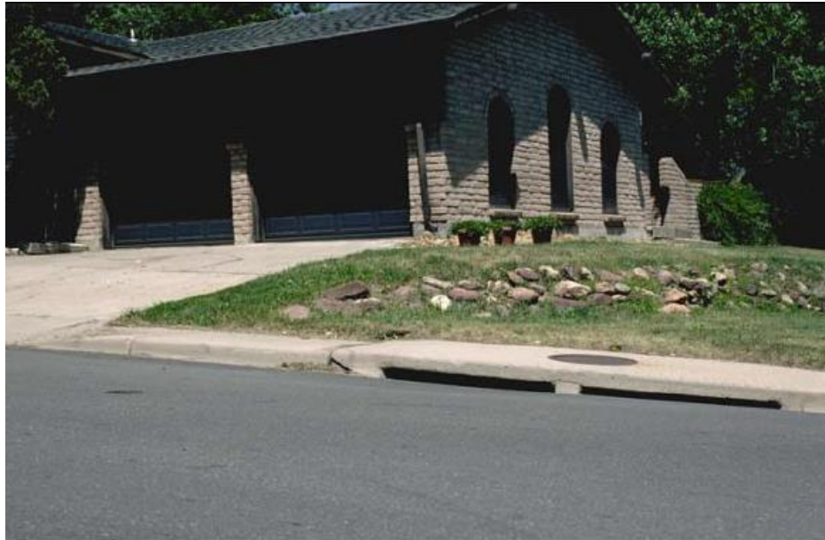
Figure 7. Depressed on-grade curb inlet with flush slab support (Denver’s Drainage Criteria Manual, Photograph ST-3, pg. ST-20).
