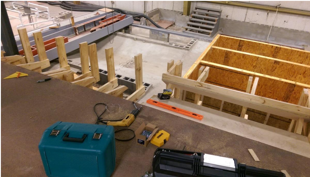
Figure 37. Photo of the 2x6 inch beams used to construct the TxDOT curb inlet.
