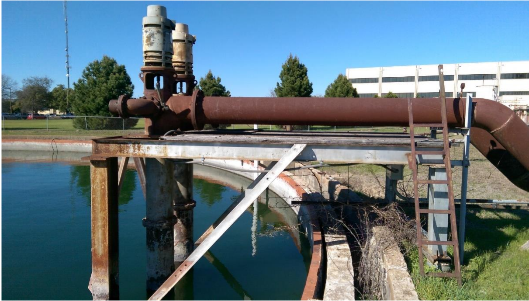
Figure 61. Photo of physical model pumps and exterior reservoir.
