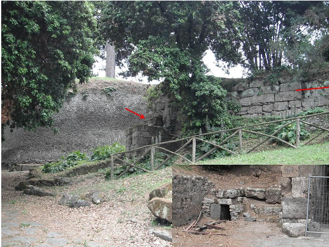
Figure 52 Porta Nola drain viewed from outside the city. The arrow marks the outlet, and the red line emphasizes the limestone/ tufa transition. The inset shows the drain inlet, photos author.
