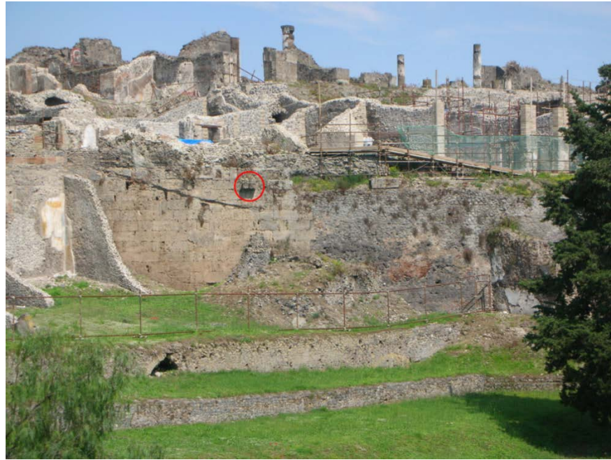
Figure 21 The limestone fortifications beneath the House of Umbricus Scaurus. The circle marks the only surviving spout. Note the opus incertum substituting the limestone to the right, photo author.
