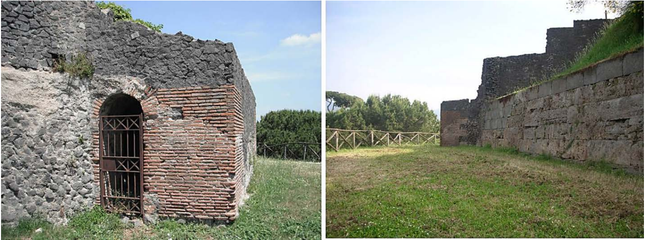
Figure 86 Brickwork on Tower V, photo author.
