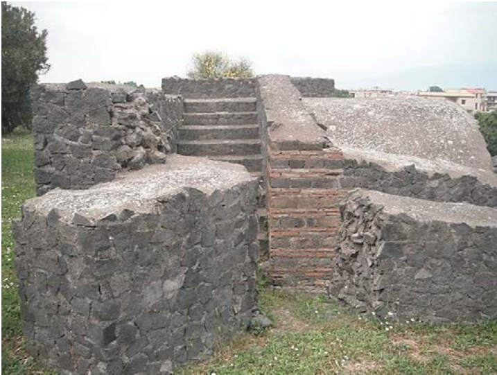
Figure 60 Tower V as part of group three. Note the variation of the staircase and the blocked off arrow slit at the end of the corridor to the postern, photos author.
