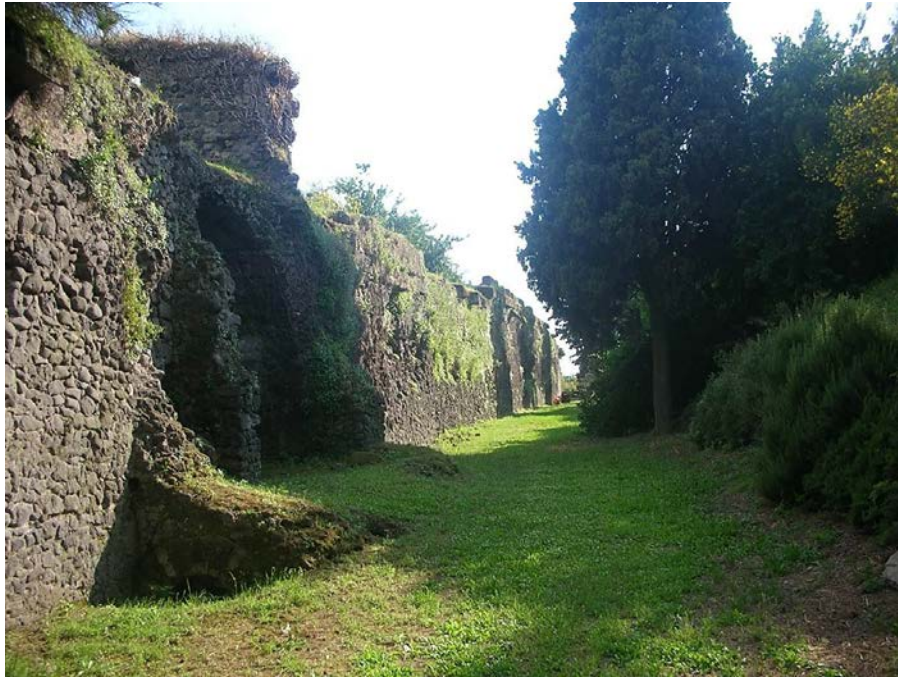
Figure 72 Opus incertum leading up to the Porta Ercolano. Note the remains of Tower XII to the left including the buried postern, photo author.
