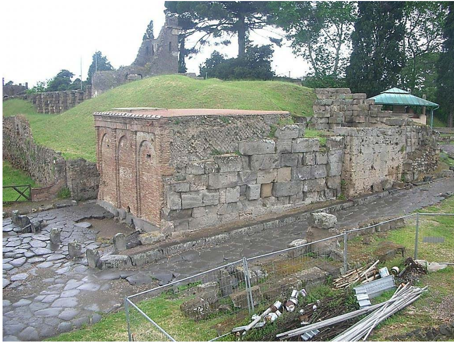
Figure 78 Overview of the Porta Vesuvio from the south east. Note the castellum cutting off the gate court wall, photo author.
