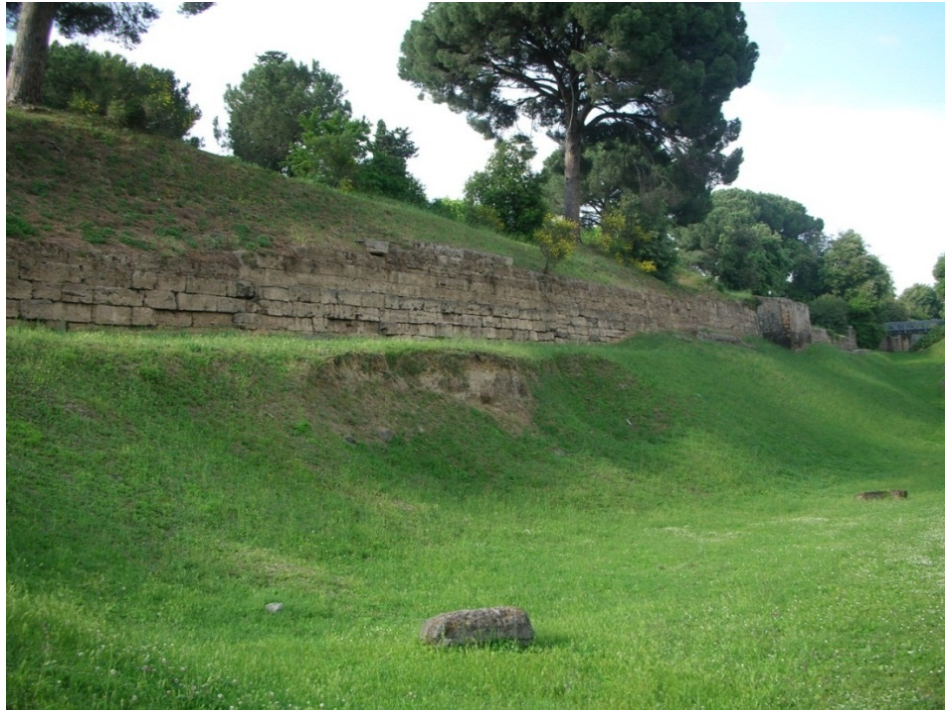
Figure 35 Wall curtain near Tower III. Note the exposed wall foundations of the lowest courses and the dark grey of the tower, photo author.
