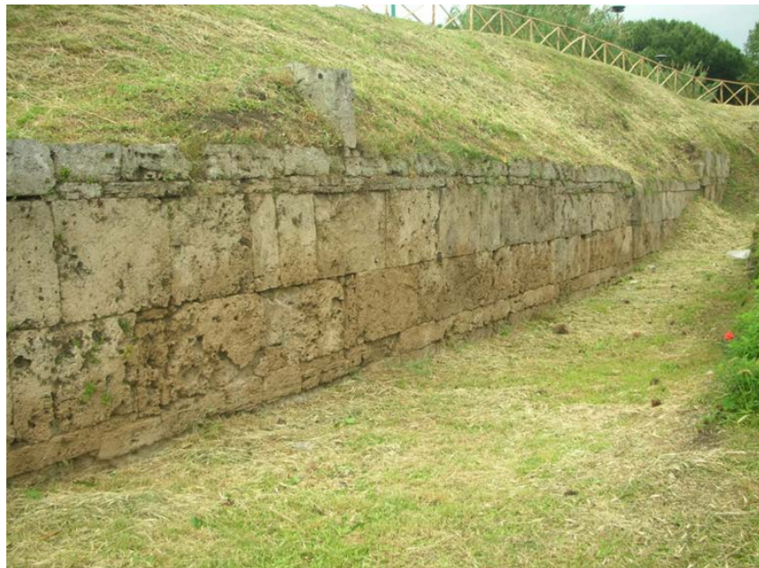
Figure 3 Remains of the orthostate wall near Porta Vesuvio, photo author.
