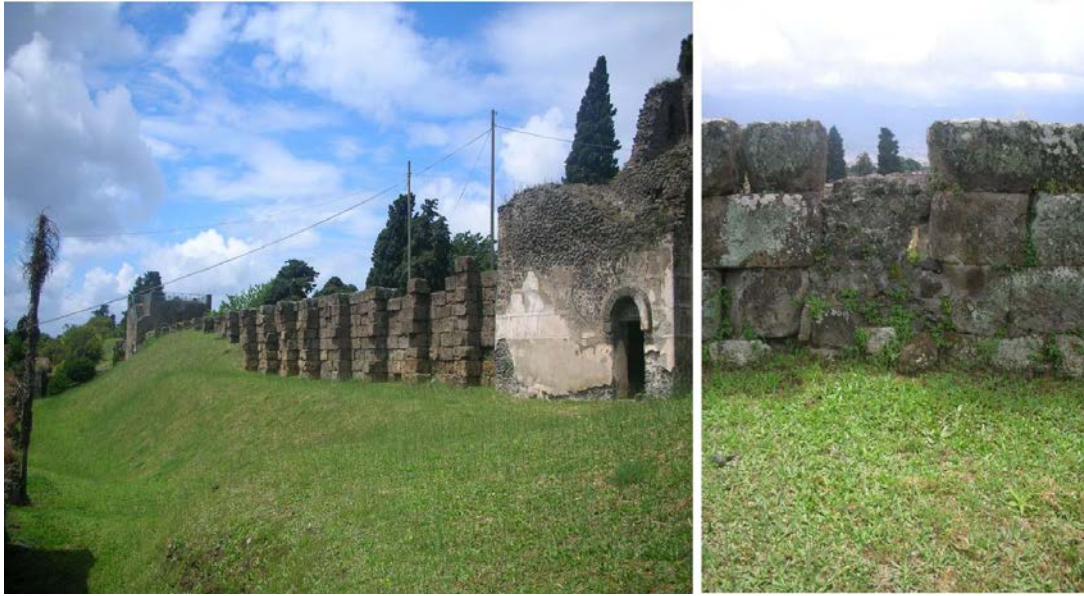
Figure 47 Lowered agger near Tower X and the walled-up postern on the right, photo author.
