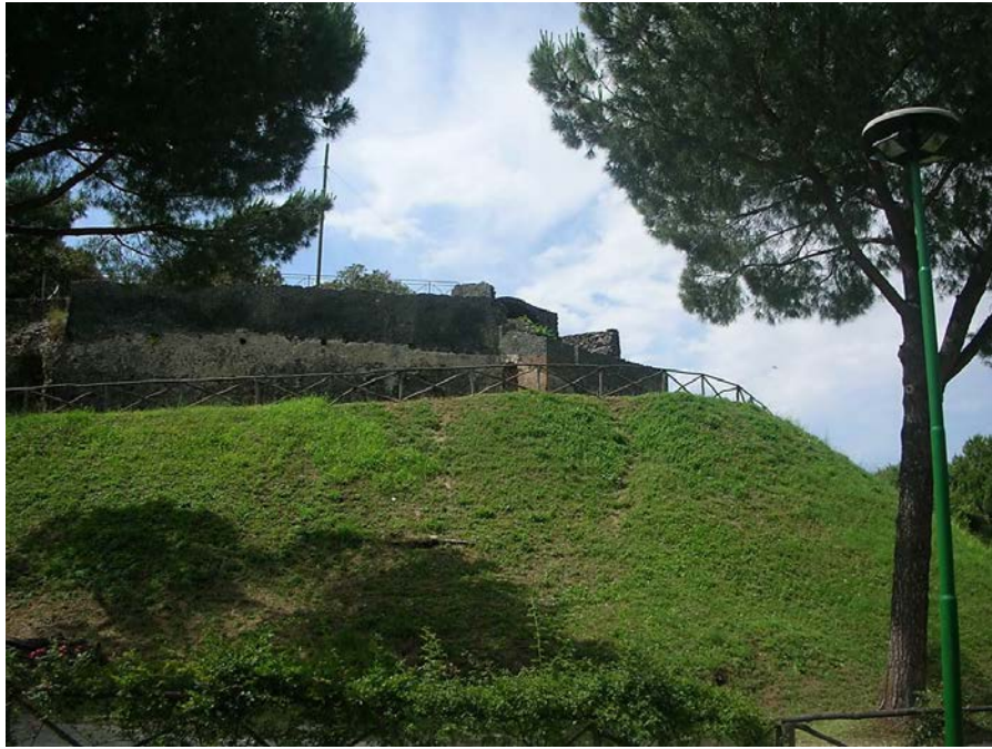
Figure 70 Opus incertum leading up to Tower V. Note the remains of stucco on the original masonry, photo author.
