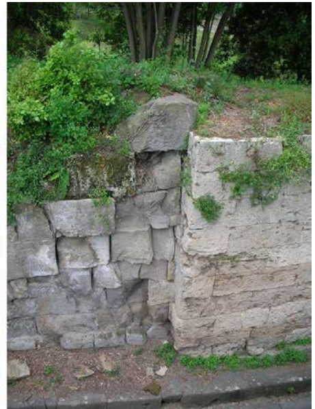
Figure 42 The gate court of the Porta Nola. Note the difference in masonry between the limestone bastions and the tufa court, photo author.
