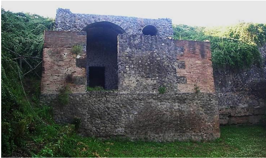
Figure 84 The Ruins of Tower II. Note the brick quoins above the exposed foundations and the rectangular openings in the front and back. The fence on the left leads to the floating postern, photo author.
