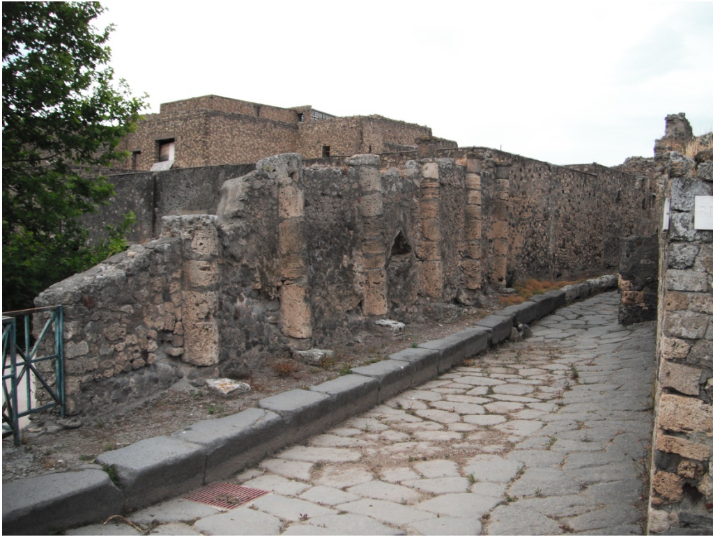
Figure 49 The columns in the vicolo dei Soprastanti. Note the central triangular opening and the drain below, photo author.
