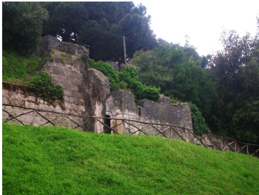
Figure 36 Tower VI near the amphitheater. Note the limestone and tufa masonry on the left and the tower clearly cutting into it, photo author.
