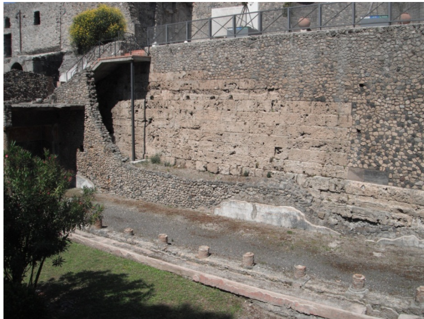
Figure 22 Remnants of the rustication in the lowest three courses south of the Porta Marina, photo author.
