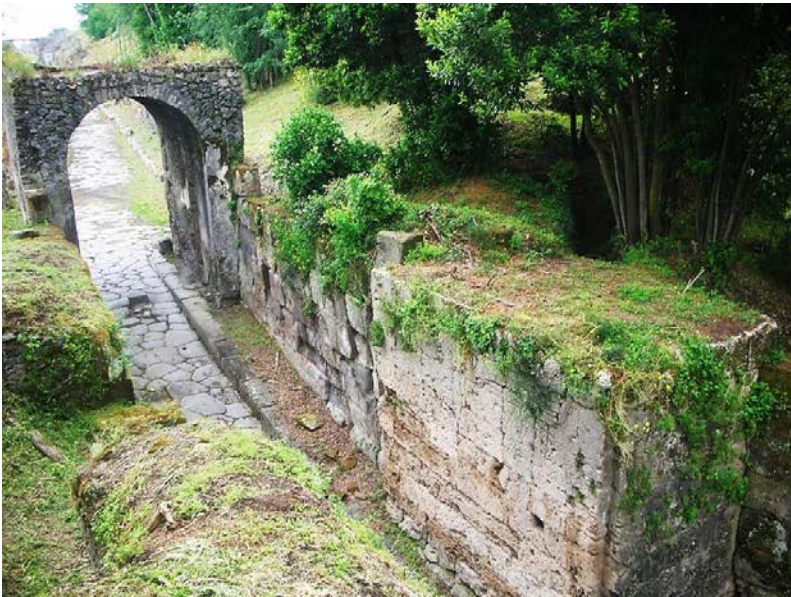
Figure 42 The gate court of the Porta Nola. Note the difference in masonry between the limestone bastions and the tufa court, photo author.
