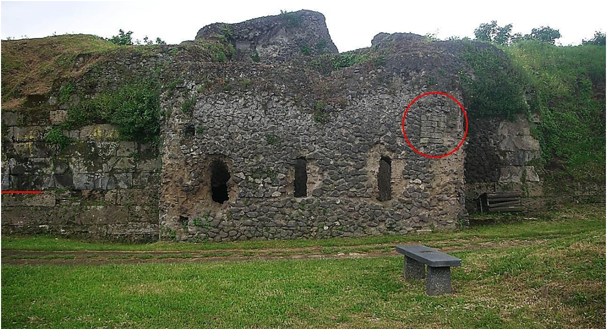
Figure 88 The ruins of Tower VII. The circle marks the opus vittatum tufa quoin. The red line marks the transition between limestone and tufa, photo author.
