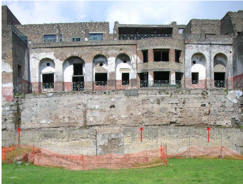
Figure 25 The fortifications beneath the House of Fabius Rufus. The three arrows indicate the seams in the wall, photo author.
