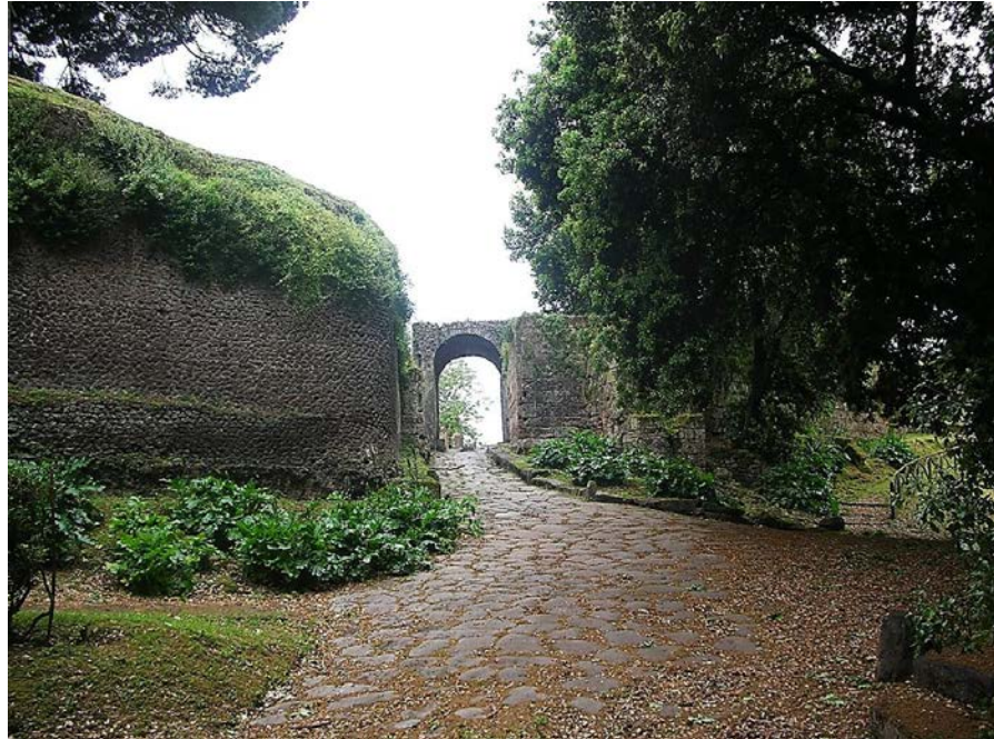
Figure 71 The Porta Nola as seen approaching the city. Note the opus incertum bastion on the left, photo author.
