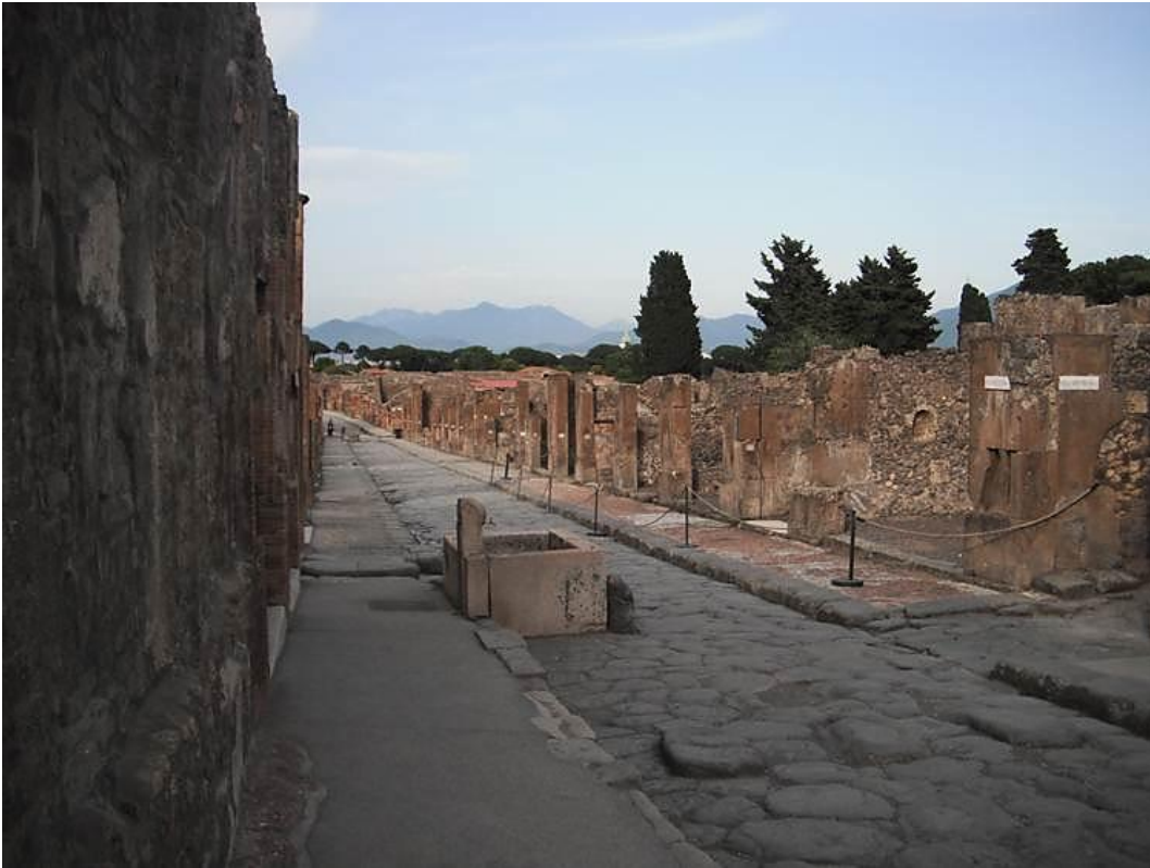
Figure 64 Tufa façades lining the via dell'Abbondanza, photo author.
