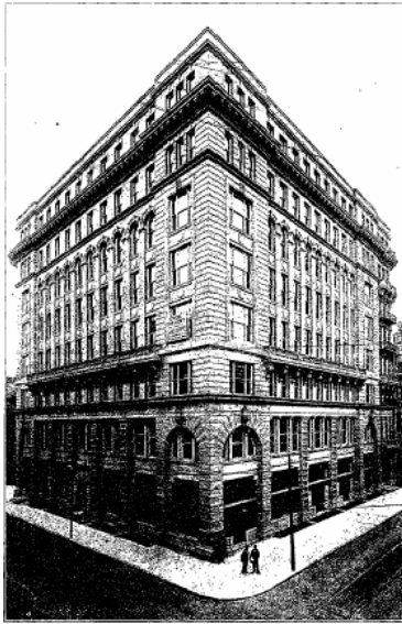
131st Street CHAS. H. BEE & CO., BANKERS JAMES H. WALTON, ARCHT. MARINER AND MERCHANT BUILDING, Chestnut Street, S. W. cor. 13d Completed amid its old neighbors, a grand substantial brick and granite office building, erected upon the original site of the old corner known as Newberry Row. Cost $400,000.
