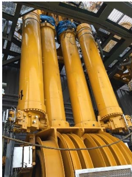
Fig. 1.4 Tensioner Cylinder and Accumulator
