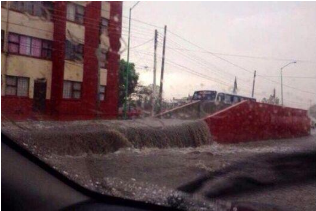
Figure A-2: "El Arenal" Drainage Channel Overflowing (Source: Evalúan daños)
