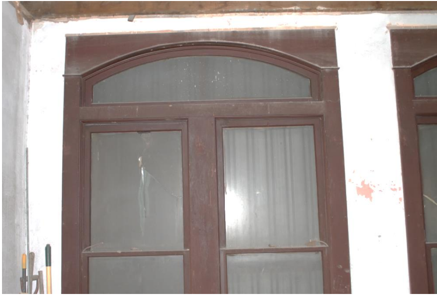
Illustration3.2: Interior shot showing metal slip cover protecting original windows
