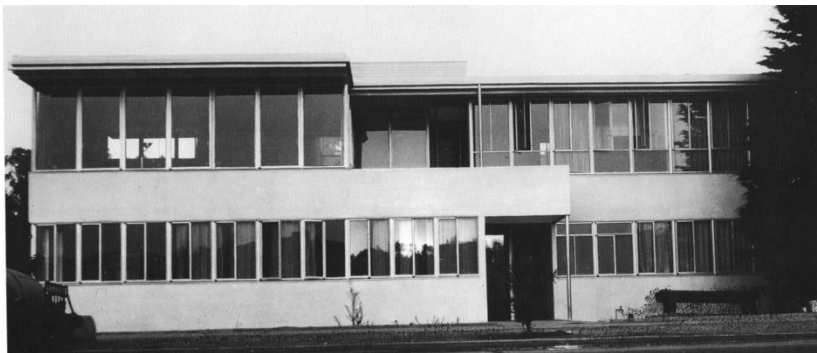
Figure 10. VDL Research House (1932). View from Silverlake Boulevard. (Hines, Architecture of the Sun , 367.)
