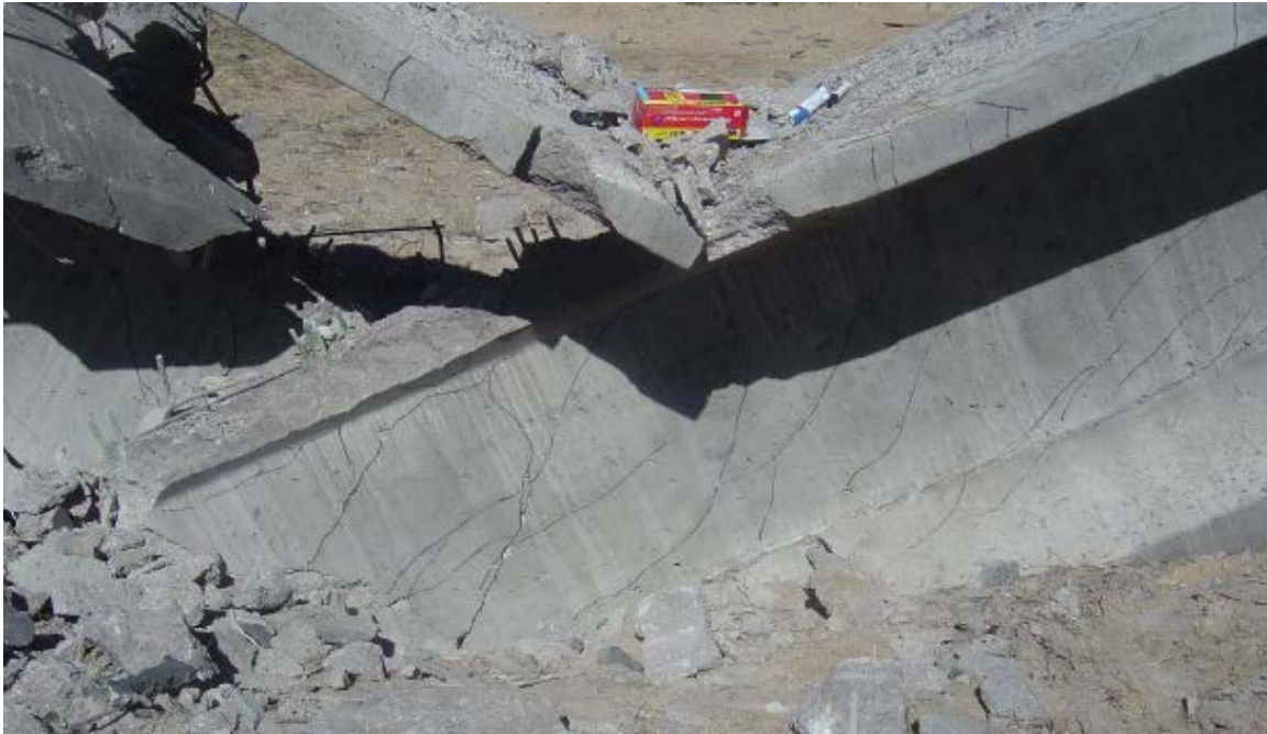
Figure 6.4: Test Specimen Below-Girder Detonation Load Case (Matthews, 2008)
