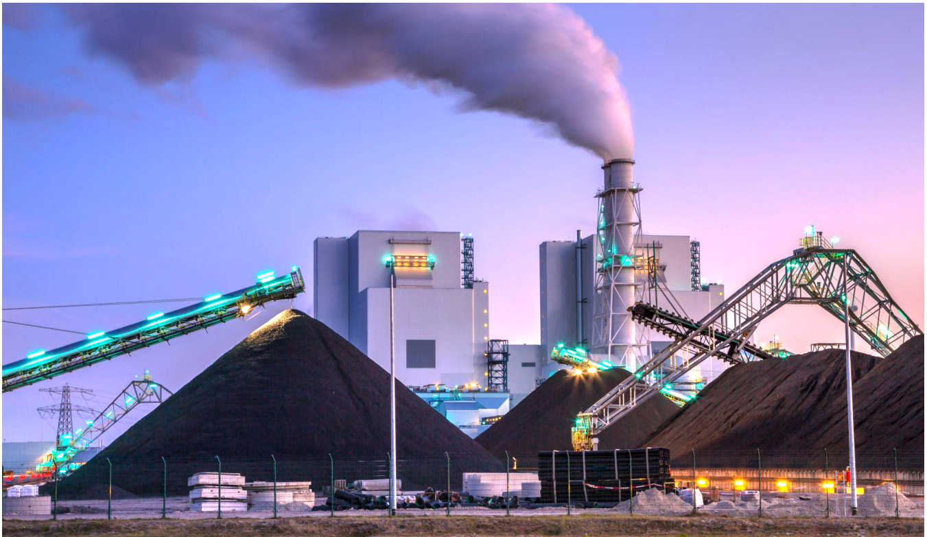
Figure 11.6. An operating coal power plant. Texas based CPS Energy has publicly expressed interest in exploring geothermal as part of a conversion project for its J.K. Spruce Power Plant, located southeast of San Antonio, Texas. Source: Stock photography.
