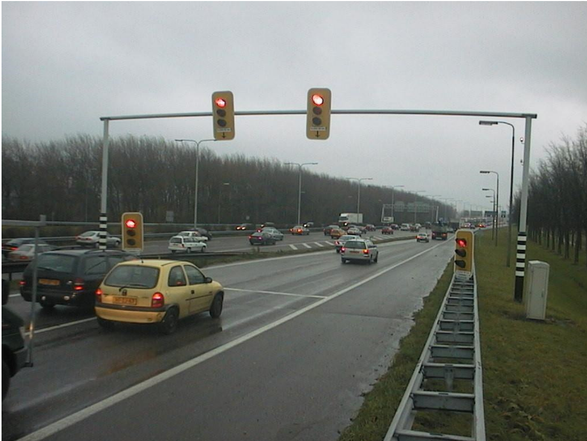
Figure 7: An example of ramp metering in The Netherlands
