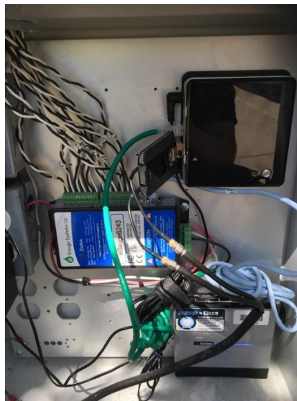
Figure 8: The installation of components adjacent to the breaker panel (early installation)
