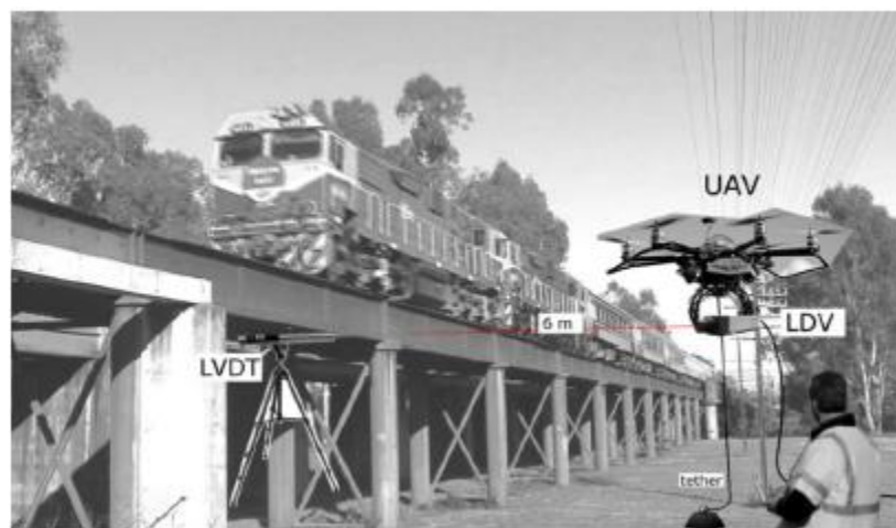
Figure 6: From [35] Tethered UAV mounted bridge displacement sensor for inspecting railway bridges under load
