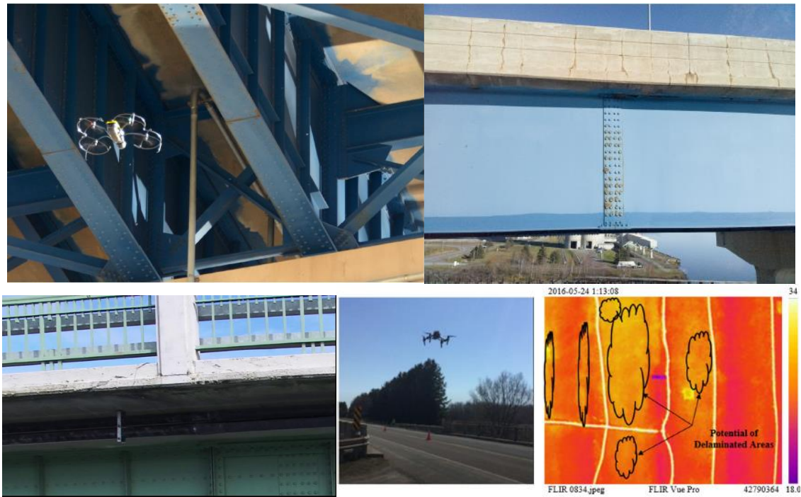
Figure 5: (top left and right) From [31], UAV mounted optical camera used for visual inspection of bridge structure. (bottom left) image from [33], shows cracking of concrete railing. (bottom right) from [34], UAV mounted IR camera for capturing delamination in bridge deck.
