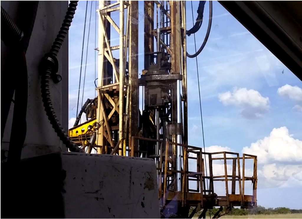
Figure 16. Snubbing jack near maximum height as it snubs out pipe.
