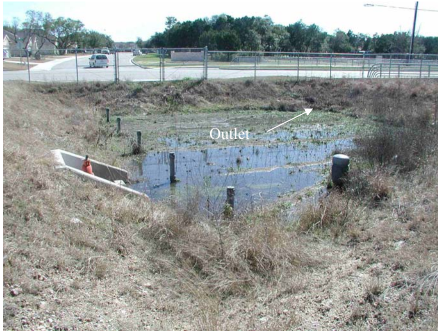
Figure 9 Photo of the Original Sand Filter Basin
