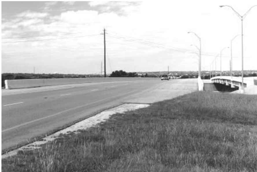
Figure 2.2 Photograph of MoPac at Convict Hill Road
